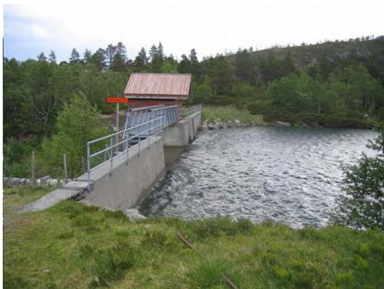
Dam Riksheimdalen (Foto: SE)
