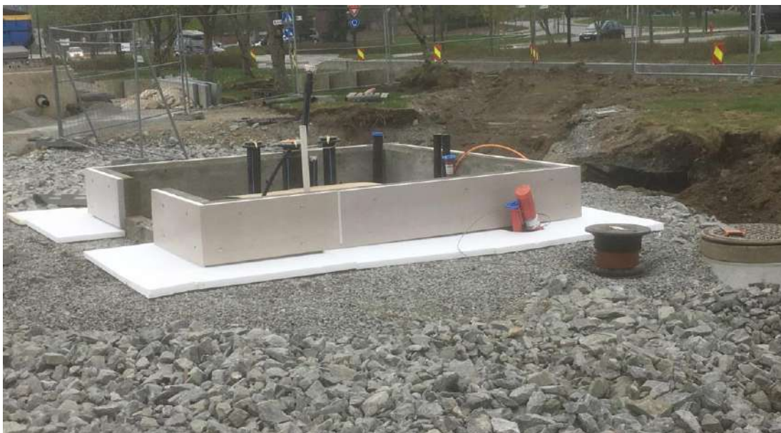
Figur 6: Ringmur pumpehus.
